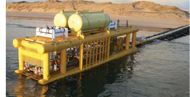
Pipeline Bundle launch
